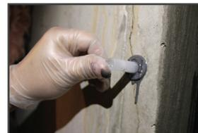
02: Press port firmly directly over crack
