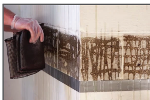
01: Mount carbon fiber to the wall
